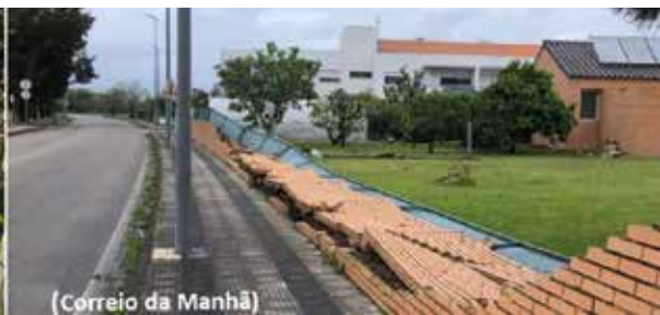
▲ Figure 8 - General view of a property wall (left), in Murtosa. Damaged wall after the strong wind event of the 08 th April 2024 (right) (photo in public circulation on the Internet).
